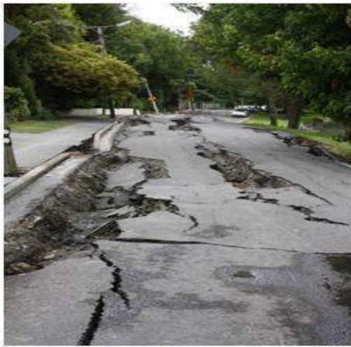
Figure No 23 Soil Liquefaction
